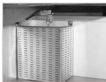
strainer on the pan outlet
